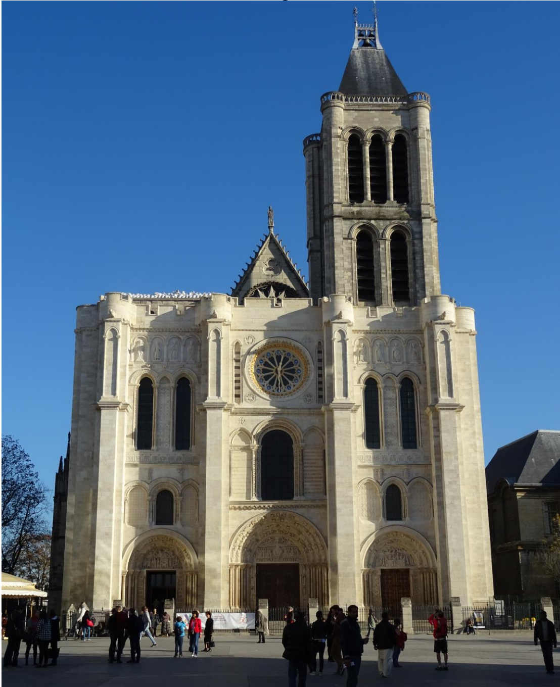
Current view of the restored western facade of the Abbey of Saint-Denis. The north tower was dismantled in 1846 due to structural problems. Photograph by the author.
